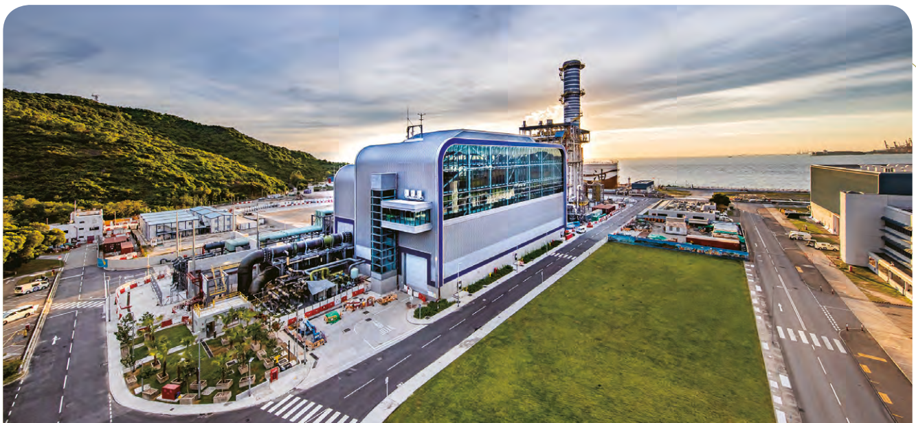
⊙ The commissioning of the CCGT unit at Black Point Power Station increased the use of natural gas to around 50% of CLP's fuel mix in Hong Kong in 2020.
